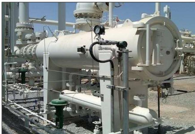
Amine Filtration coalescing and filtration systems allow for optimized performance of the downstream heat exchanger and amine regenerator section. Rich amine coalescing and filtration systems impart the following benefits to the unit:
